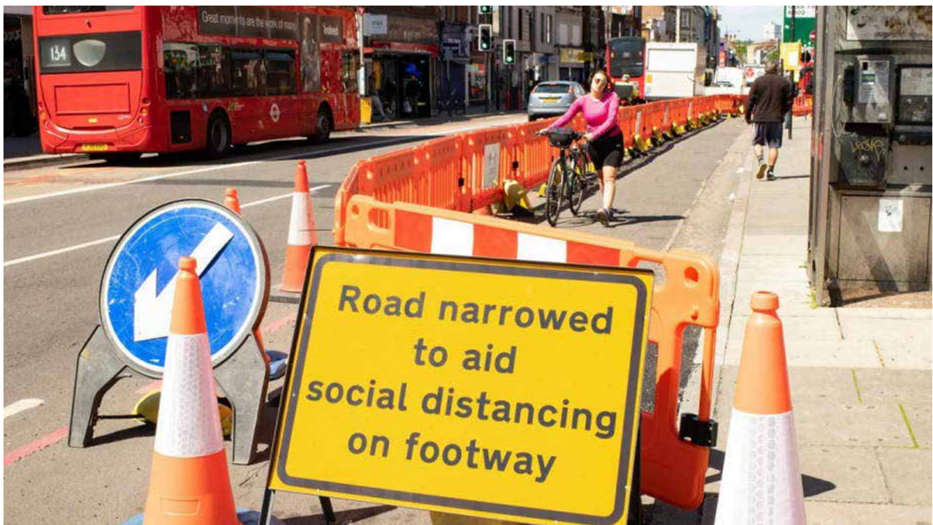
Street re-allocation to ensure social distancing in London
